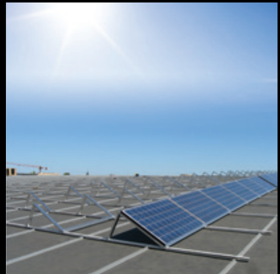
Industrial building (Belgium)
