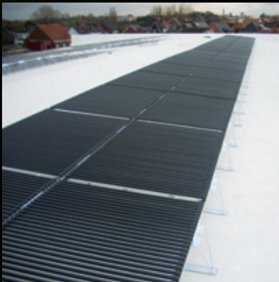
Industrial building (Belgium)
