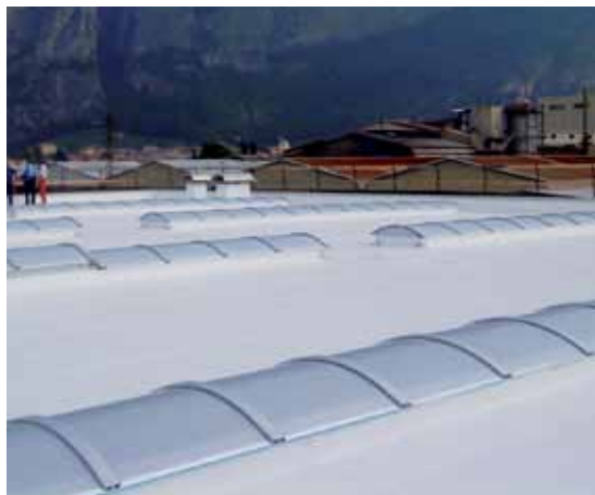
Industrial Building (Italy): RENOLIT ALKORBRIGHT
