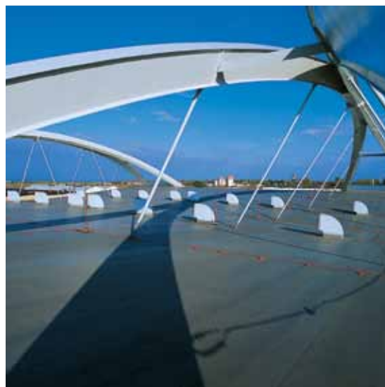
Transport station (Czech Republic)
