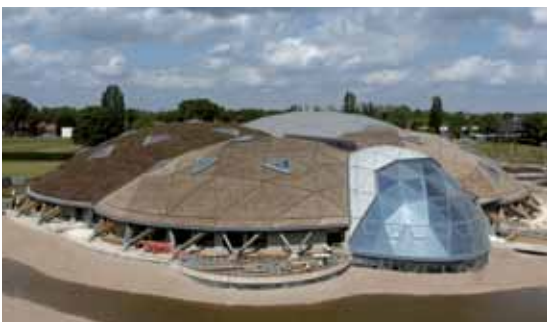
Scunthorpe Leisure Academy (UK)
