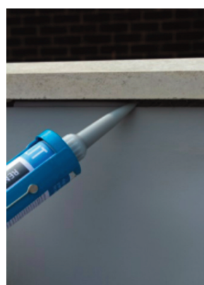
Sealing perimeter upstand
