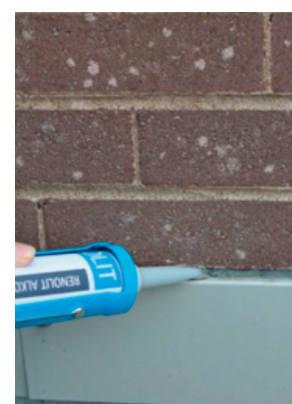
Sealing chased metal edge to RENOLIT ALKORPLAN onto a sacrificial layer
