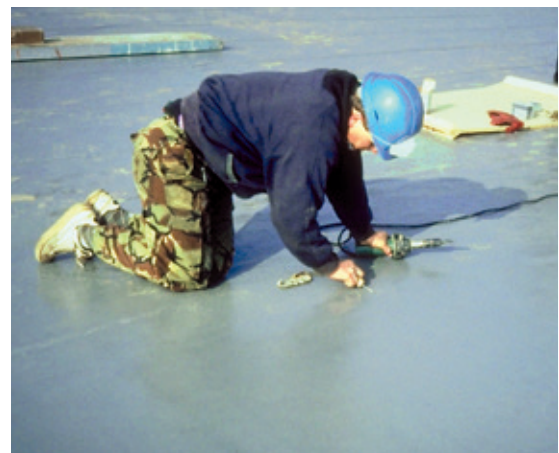
fig. 2: Verification of weld security
