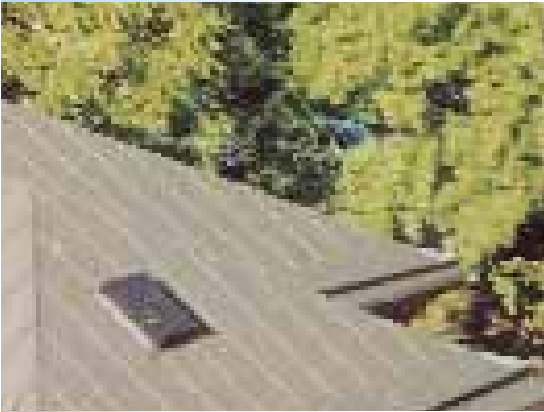
Project: Doctor's private cabinet and psychiatric hospital Stockholm, Sweden, 2000 Product: AlkorDesign (150 sqm) Old waterproofing: zinc
