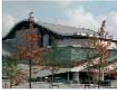
Project: Classé Theatre (Breda, The Netherlands, 2002) Product: AlkorPlan® F (Mechanical fastening, 1,500 sqm) Old waterproofing: Synthetic
