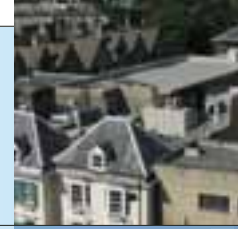
Project: Blackwells Library (Oxford, UK, 2003) Product: AlkorPlan® F (Mechanical fastening, 300 sqm) Old waterproofing: bitumen
