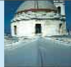
Project: Bari Cathedral (Bari, Italy, 1980) Product: AlkorPlan® Mechanical (Adhesive, 2,000 sqm) Old waterproofing: bitumen
