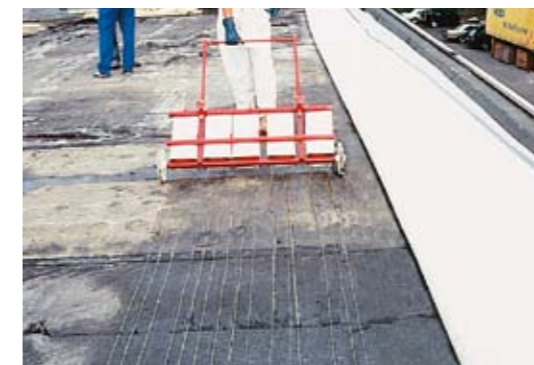
Pict. 1 use of the alkorPLUS ® 81069 Applicator When the adhesive is applied in lines, as illustrated, it must be squeegeed across the width of the membrane to create a full bond.
