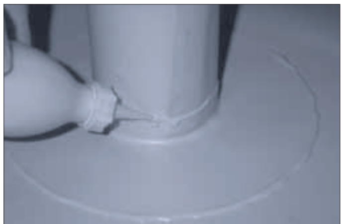
Fig. 3: Liquid ALKORFLEX® 81036 applied with the ALKORPLUS 81145 PE bottle and nozzle 81245
