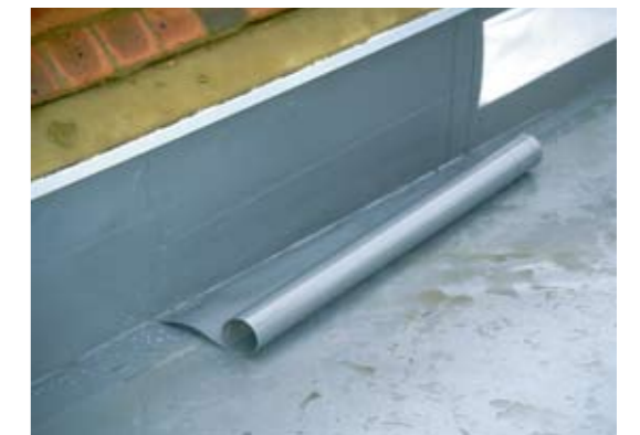
Fig. 3: Edge restraint with alkorPLUS ® 81170 metalsheet
