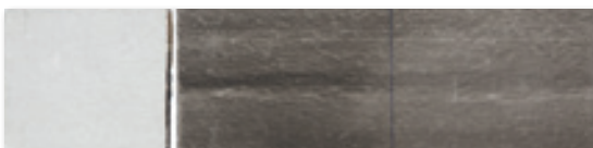
Bitumen roofing membrane with a smooth, reflective acrylic coating on top
