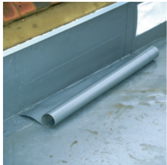
Fig. 3: Edge restraint with RENOLIT ALKORPLAN 81170 metalsheet
