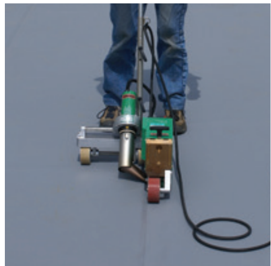
Using a hot-air welding machine
