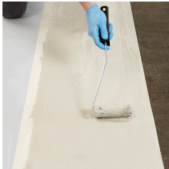
Sealing of the connection between PVC-waterproofing and bituminous waterproofing
