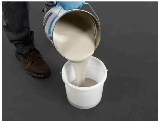
2. Decide the amount of resin or primer needed. Do not mix more material than the quantity that can be installed within the curing time.
